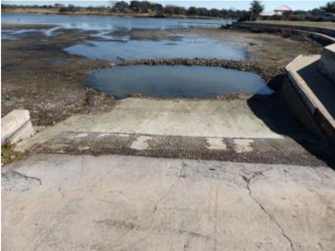
New grate on the boat ramp at Dove Park
