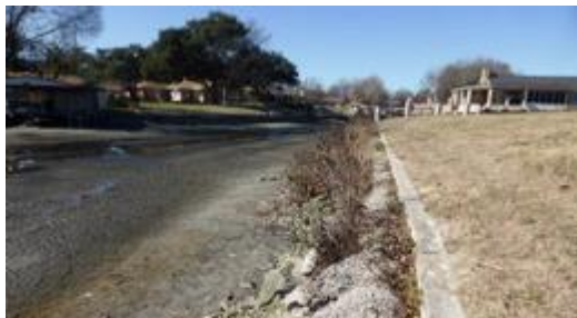
Work on the retaining wall
